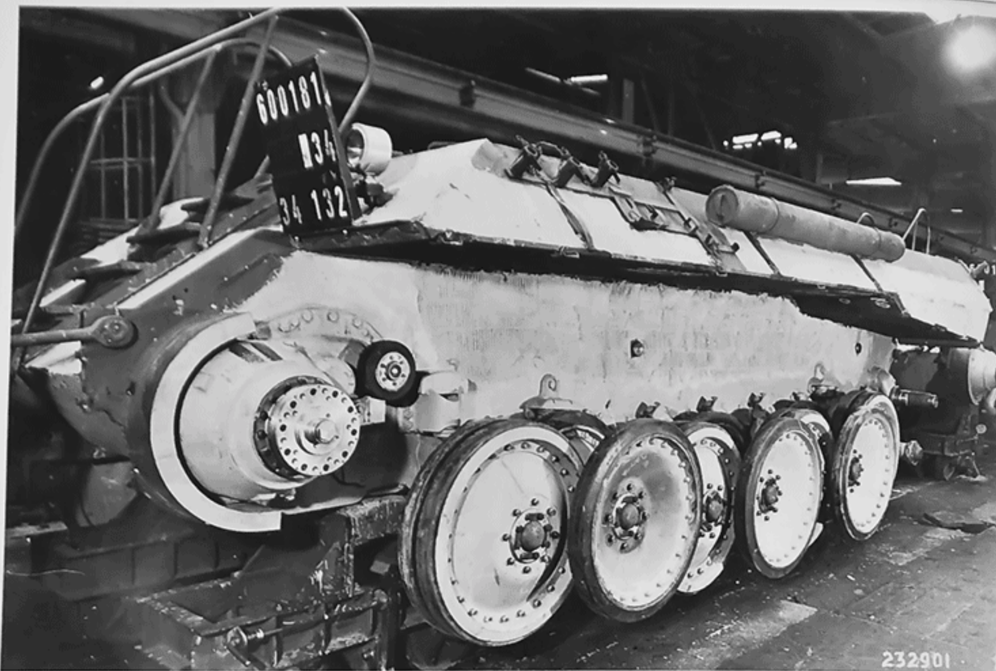
Panther Ausf. A in the assembly line at M.A.N., Nuernberg in January 1943. Mounted on wheeled trucks on a rail line, the chassis moved along the assembly line from station to station. (CHY)
