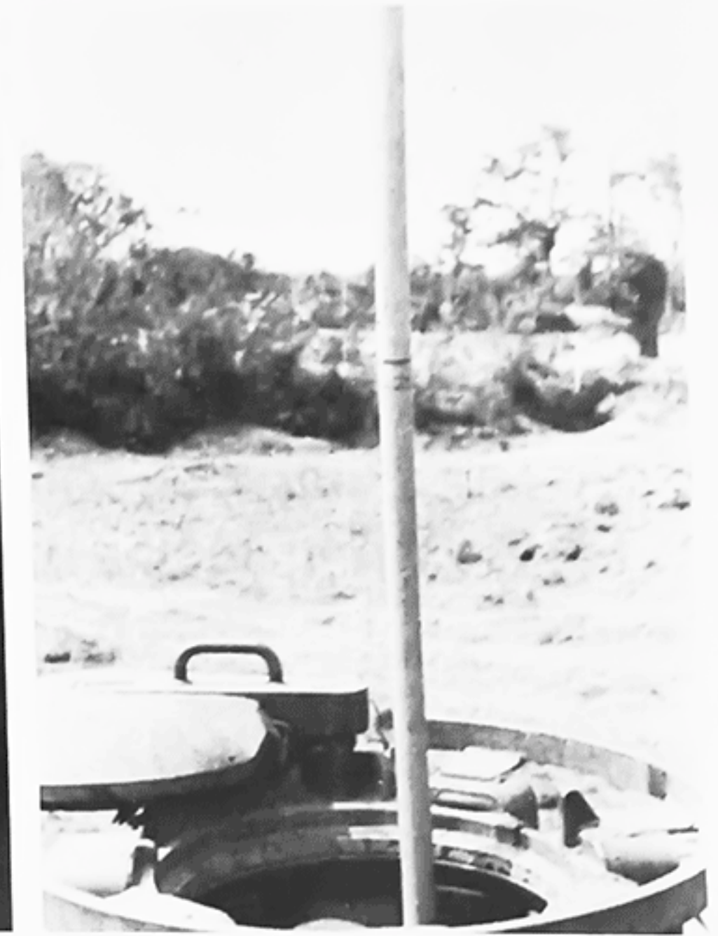
T.S.R.1 Sehstab (periscope) mounted in the turret allowed the commander to reconnoitre from turret-down positions. (HLD)
