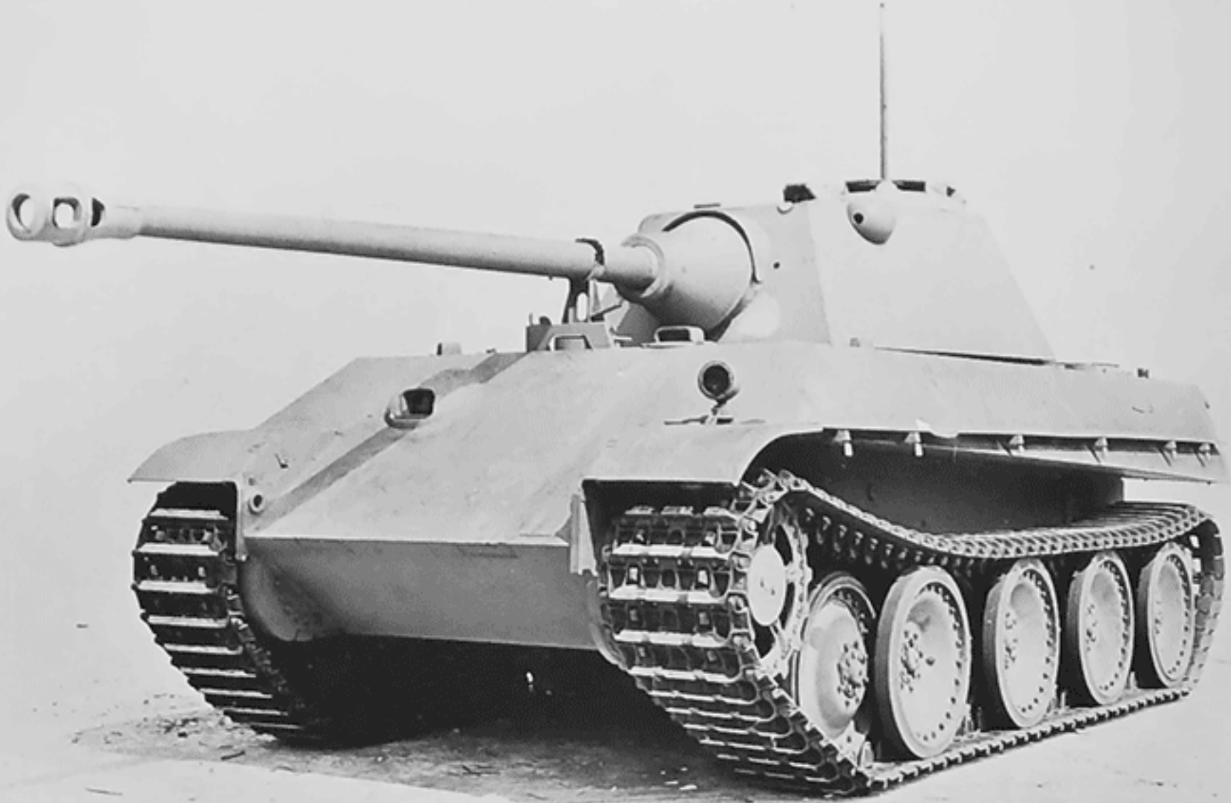
Above and opposite above: A Versuchs-Schmalturm (experimental narrow turret) mounted on a Panther Ausf.G chassis manufactured for Wa Pruef 6 (no tool or equipment stowage). These photographs dated 20 August 1944 reveal that experimental work had proceeded on the Schmalturm at a much earlier date than previously thought. An aperture for a "monocular" gun sight (not the binocular T.Z.F.13 ) has been drilled in the turret front. A periscopic gun sight is mounted in the left front turret roof. The redesigned commander's cupola had a hole for extending the T.S.R.1 observation periscope without opening the hatch. (BA)
