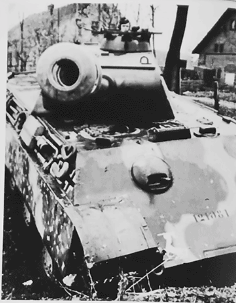
Panther Ausf. G (Fgst.Nr. 121081 completed at M.A.N. in late September 1944) was issued to I.Abteilung/Panzer-Regiment "Hermann Goering." Zimmerit was not applied and patches of camouflage paint were sparingly applied to the red oxide primer base coat. (JW)
