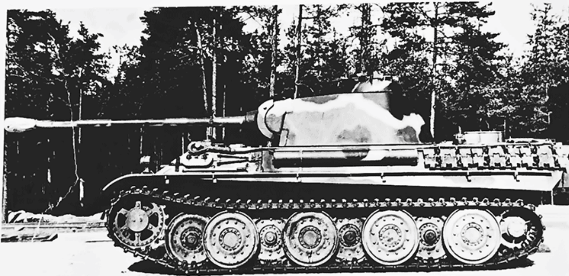
One of the small series of Panther Ausf. Gs (Fgst. Nr. 121052 completed by M.A.N. on or about 22 September 1944) outfitted with steel tyred roadwheels. These roadwheels were the same type used on the Tiger I and Tiger II but were mounted in the normal Panther pattern running on normal Panther tracks. By the time this Panther was completed Zimmerit anti-magnetic coating was no longer being applied. A rain guard has been fitted over the driver's visor. The fan tower on the rear deck was backfitted to this Panther. (NA)
