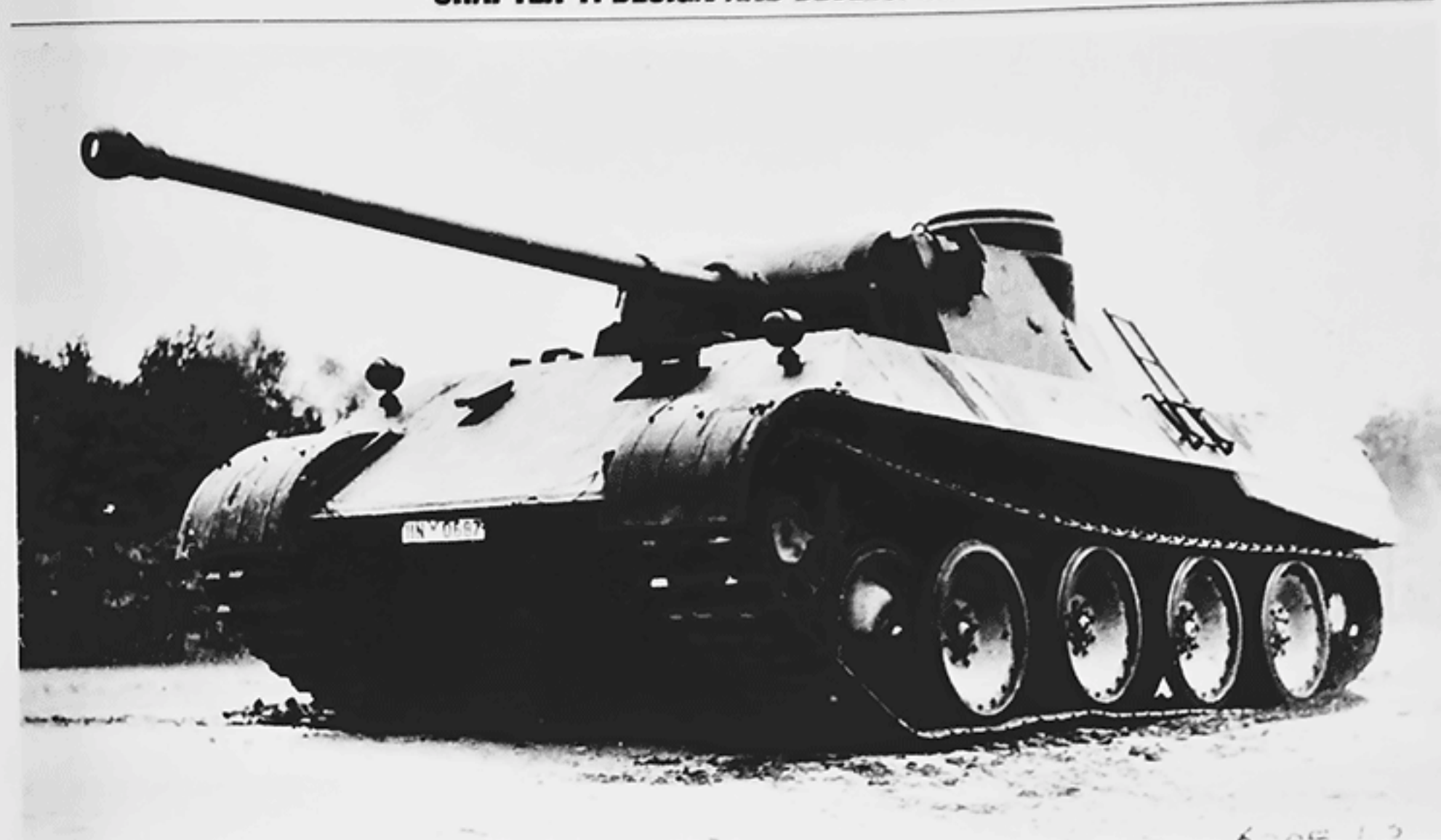
Versuchs-Panther (Fgst.Nr. V2) completed by M.A.N. in the Fall of 1942) was outfitted with a turret. The 7,5 cm Kw.K.42 L/70 still had the ball muzzle brake invented for the 7,5 cm Kw.K.40 L/43 in the Pz.Kpfw.IV Ausf.F2. (WJS)
