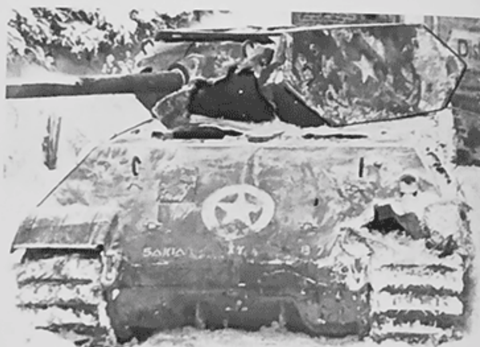
Above and opposite below: Five Ausf.G Panthers were disguised as American M-10 Tank Destroyers and issued to Panzer-Brigade 150 for the Ardennes Offensive. The M-10 silhouette was created by welding on sheet metal strips cut to shape. A flat-hinged two piece hatch replaced the commander's cupola. (CHY)
